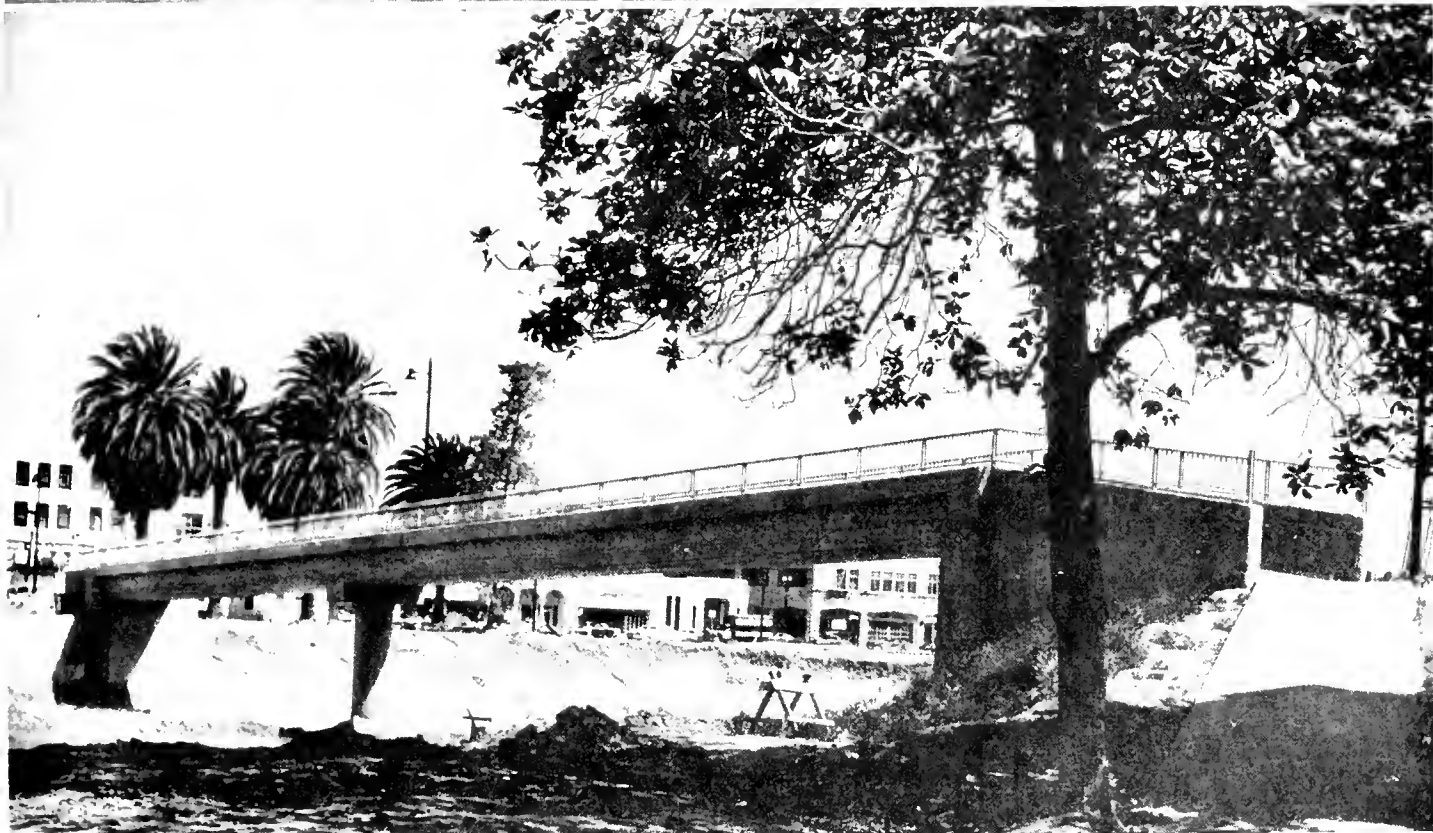
UPPER—Looking easterly along Washington Boulevard showing nearly completed underpass bridge structure carrying the Harbor Freeway. LOWER—Looking southeasterly, showing Harbor Freeway in vicinity of 21st Street, construction details of pedestrian overcrossing.
